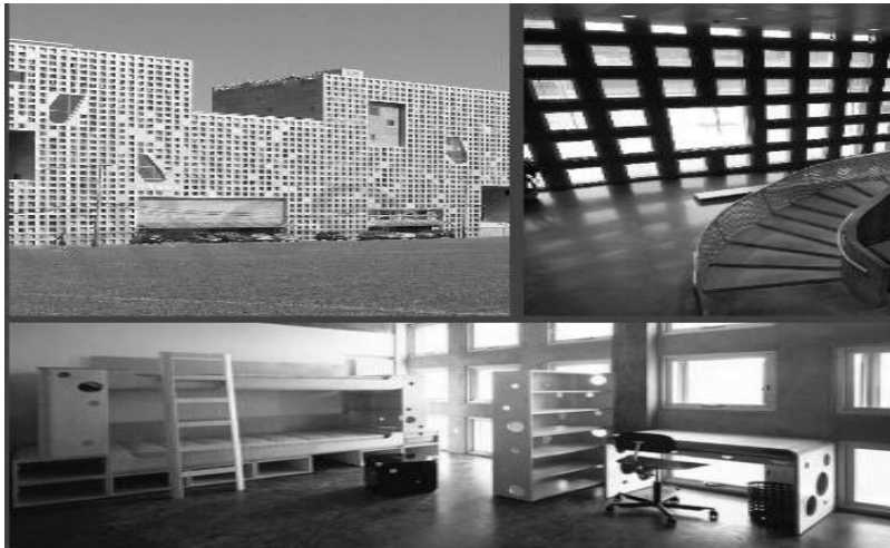
Fig. 2. The dormitories of MIT.
